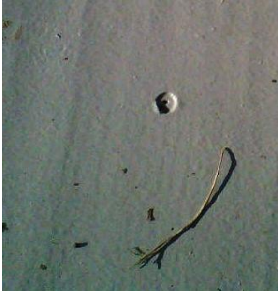
Damage done by push pins
